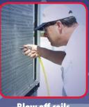
Blow off coils with Sludge Sucker® Blowgun
