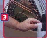
**3. Replace PVC** cap on "T" connection For future service: **DO NOT GLUE** PERMANENTLY.
