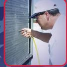
**Blow off coils** with Sludge Sucker® Blowgun
