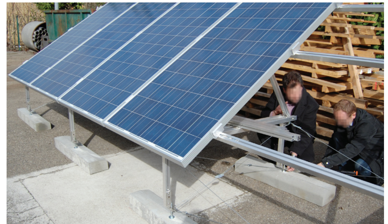
Solar Panel Installation
