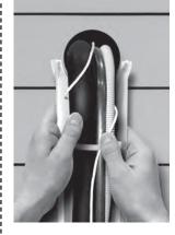
(4) Run lineset, drainhose. wiring etc. over the fitting and duct bases and secure to duct clips using tie wraps of sufficient size.
