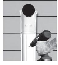
(2) Once all fitting bases are secured to the siding, measure and cut LD Ducting to fit as needed. Remember to account for some seasonal expansion and contraction. Install and fasten LD Ducting bases. Attach bases only to structure through provided punch outs using fasteners of sufficient length (not provided).
