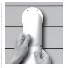
(5) Snap straight duct top over mating straight base pieces. Seat fitting tops over mating fitting bases and secure with provided stainless screws. Duct must terminate with a fitting to prevent cover from sliding out of position. If duct is to be painted, or duct is a dark color, adhere cover to base with pvc cement.
