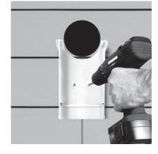
(1) Determine the path which the lineset will follow and strike a chalk line to mark the surface material. Attach the base only of all fittings first (ducting will be placed last), along the marked path, using fasteners of sufficient length (not provided). Predrill where necessary. Duct must terminate with a fitting to prevent cover from sliding out of position.
