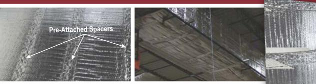
**rFOIL**<sup>®</sup> BIG-6 Reflective Duct Insulation is a 5/16" layer of polyethylene bubble, bonded to and sandwiched between two radiant barrier sheets. Then, four strips of spacers are pre-attached and run along the full length of the roll. these spacers help provide the necessary airspace to achieve an R-6.0 insulating value.
