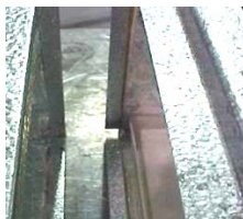
Blower Section (left) and top of coil (right) with 3/4" slot.
