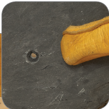
Clean recessed nail holes (as shown)
