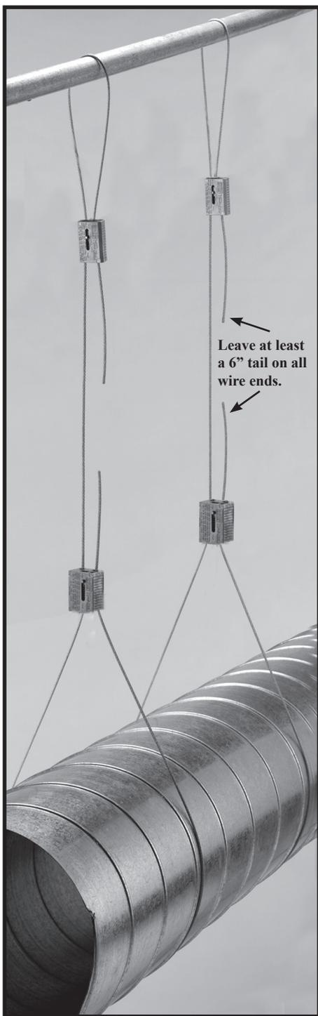
As a matter of sound engineering practice, the Dyna-Tite assembly must be located no closer than 12 inches to the suspension point. In the case of round duct, where the wire rope encircles the duct, the Dyna-Tite must be located the distance of one diameter from the duct wall.
